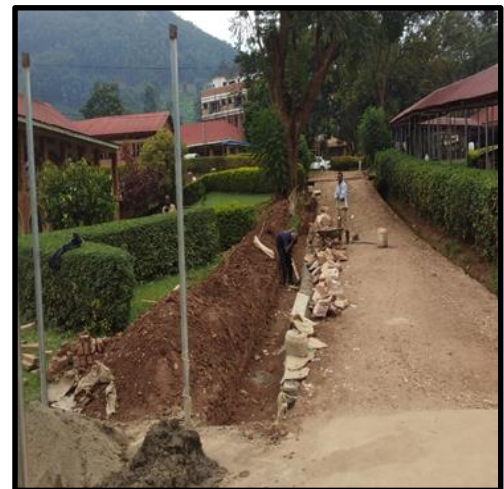
A small drainage trench being built.
