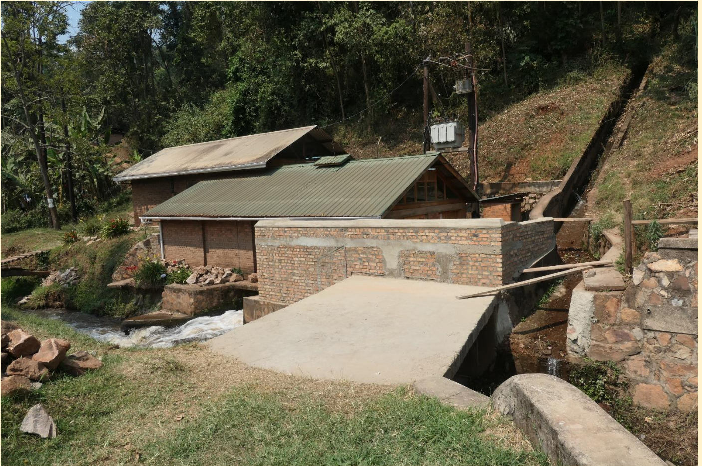
The wall around the Generator House to prevent damage from flooding... this bend has now been opened up to stop the bottleneck.
